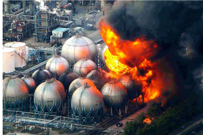
2011 TOHOKU EARTHQUAKE – CHIBA REFINERY
