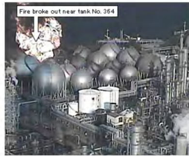
*4. Leaked LPG caught fire. (Please refer the point where the fire broke out in the image shown in the layout of the tank area*2 on the previous page.)
